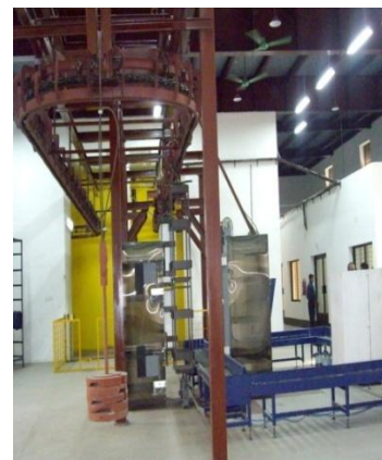
Gamma Radiation Facility at AERE
